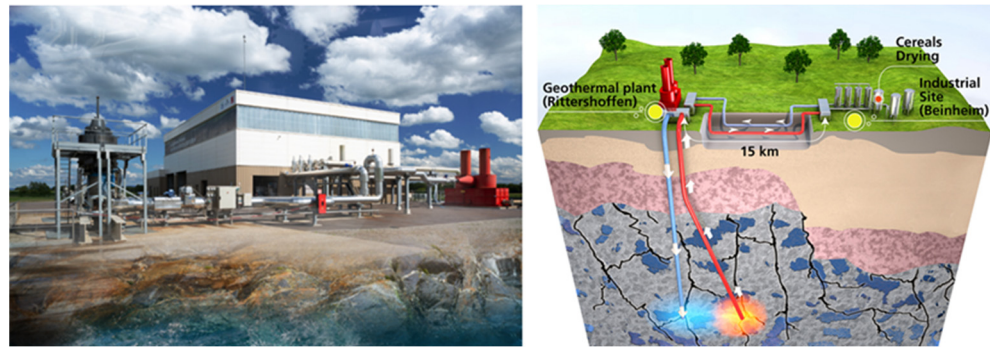
Figure 1. View of the Rittershoffen geothermal plant and schematic representation of the plant supplying heat to the industrial user (credits: ES group).
