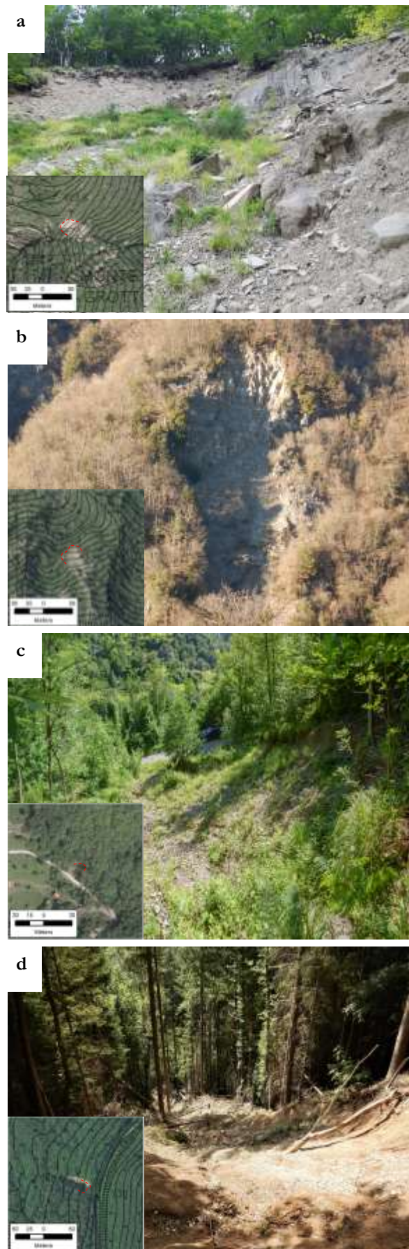
Figure 4-4 Examples of some visited landslides recognized in the study area. a-Avalanche (BR, near Chiozza). b-Fall (BR, near Castelnuovo Garfagnana). c-Planar slide (SD, near Piritano). d-Flowslide (SD, near Eglio)
