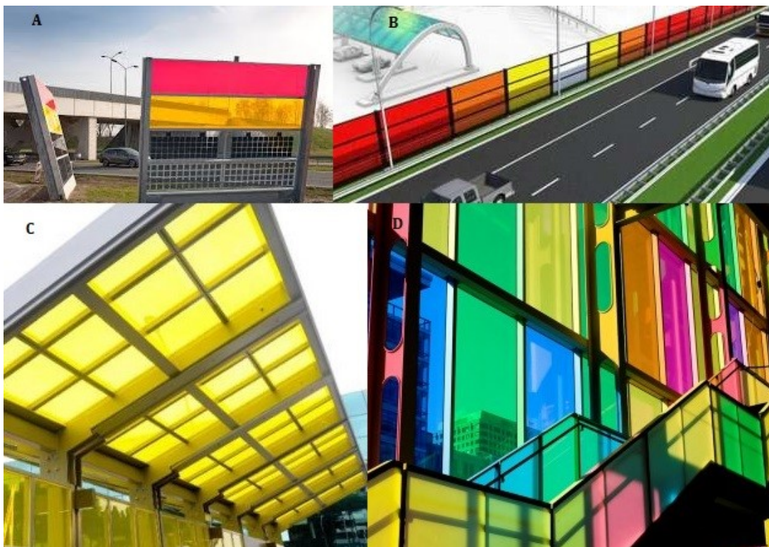
Fig. 26: BIPVs LSC-based, realized in large scale or prototypes: LSCs could be integrated in common buildings such as windows ( D : Congress palace of Montreal, Canada), penciline ( C : penciline from Eni) and sound barriers in prototype design ( A ) and in a prospective application on trunk roads ( B ) in Netherlands 117 .
