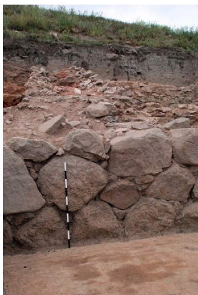
Fig. 30: The southern wall in granitic boulders of the Building III. From south
