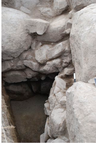
Fig. 12: A detail of the foundation structures: the row of large boulder laying on three rows of middle-sized stones (room 127, square J19 C4). From east
