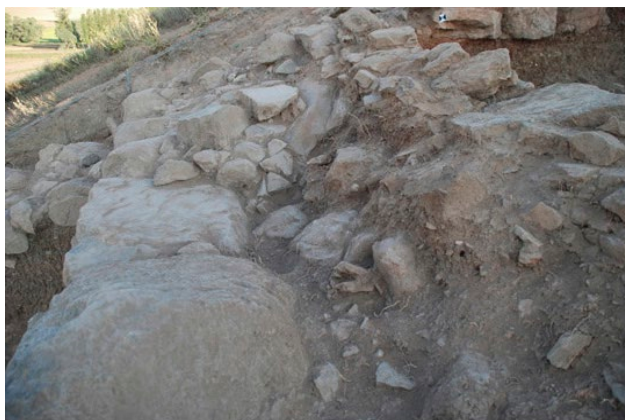
Fig. 37: Detail of the foundation wall laying on top of the boulders of the southern retaining wall 8. From east
