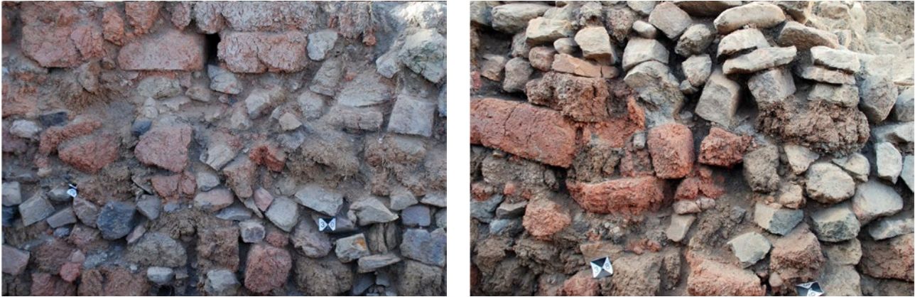
Fig. 53: A detail with the structure of the wall 31, with stones and fragmentary burned mud-bricks, without mortar. From south
