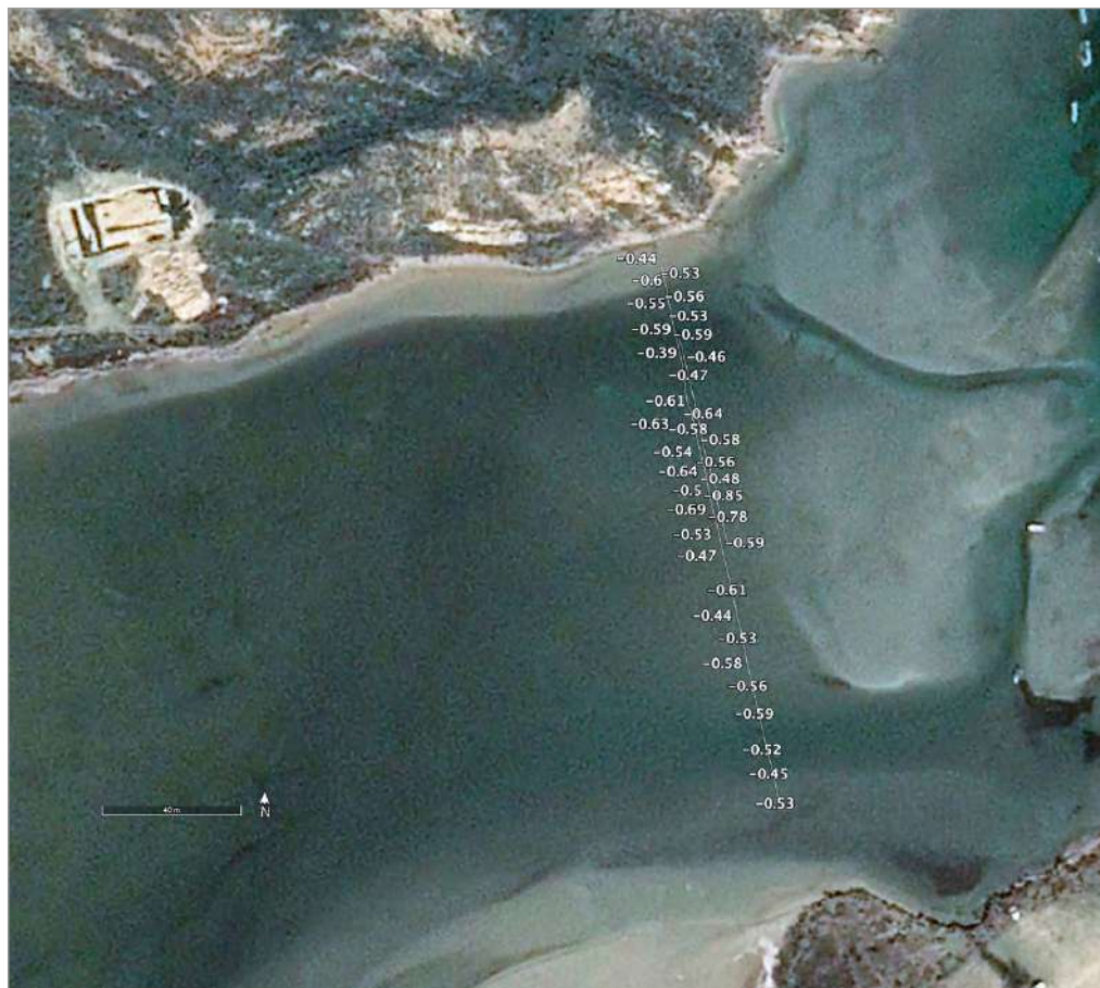
Fig. 55. Mesohaline Lagoon of Hephaestia. Elevated plan (with respect to the depth of the lagoon) with the rough positioning of the limits of the long wall on a Google Earth satellite photo (el. F. Morfea; © Archivio fotografico SAIA U/13392).
