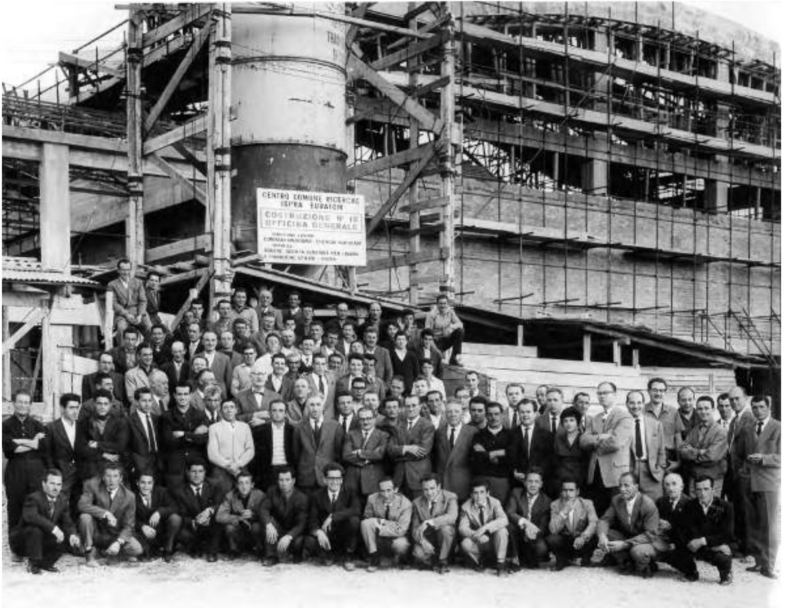
Personnel in front of the general workshop during construction, 1962.
