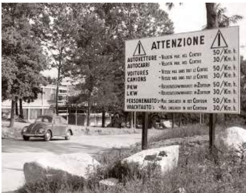
The entrance to the JRC site in the early 1960s – road sign at the entrance to the centre.
