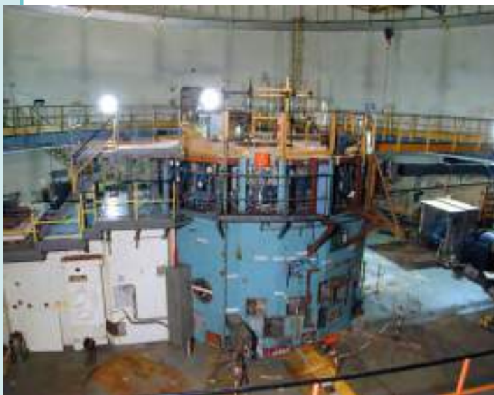
The Ispra-1 reactor interior before dismantling.
