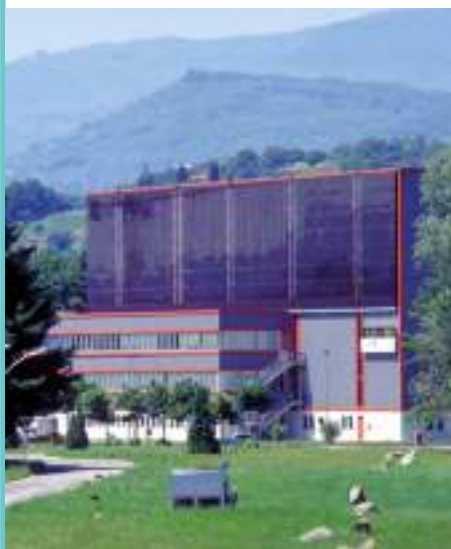
Photovoltaic panels on the ELSA building's southern façade.
