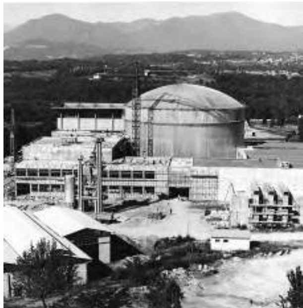
The ESSOR reactor under construction, 1965.
