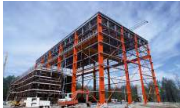
View of the ELSA building under construction, 1991.
