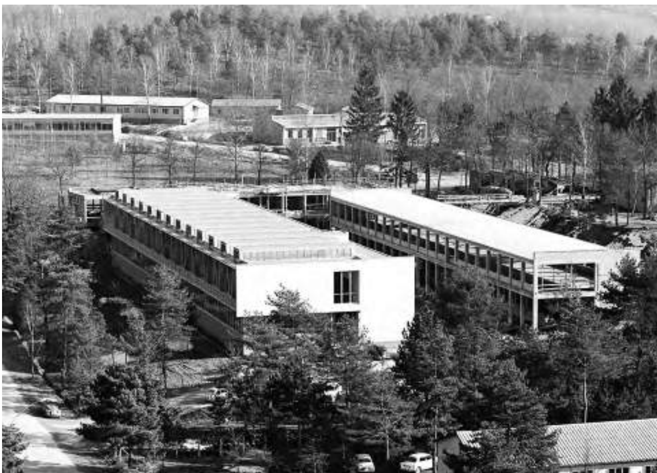
The Scientific Information Processing Centre (CETIS) building, 1962.
