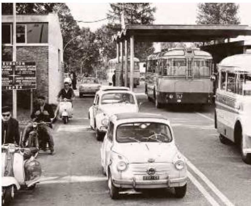
The entrance to the JRC site in the early 1960s – incoming and outgoing vehicles.
