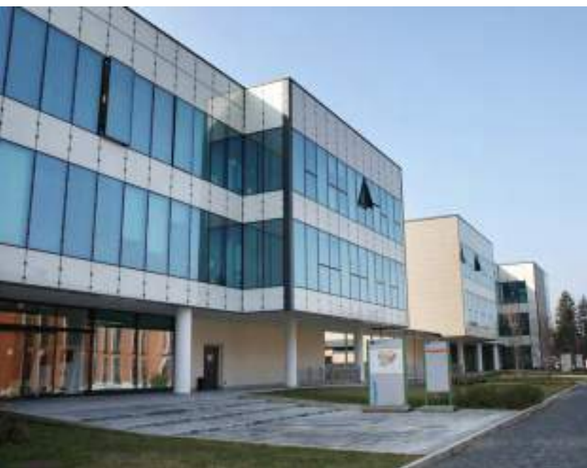
The science zone, completed project, 2017.
