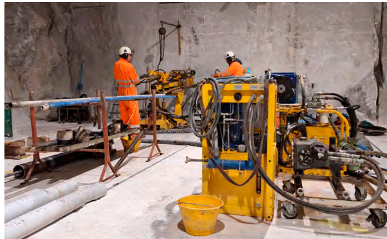
Figure 6. Stages of a sub-horizontal borehole drilling.
