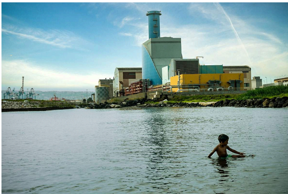
Figure 3. Napoli-Levante combined-cycle power plant within the Site of National Interest "Napoli Orientale." The scene illustrates the everyday coexistence of industrial facilities and urban life.
