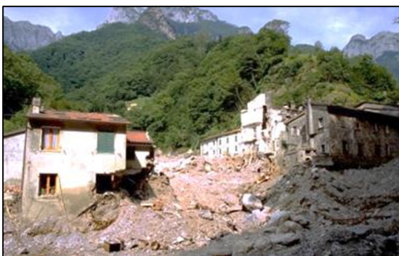
Fig. 2. Destruction of the Cardoso village caused by severe debris flows deposition [16].
