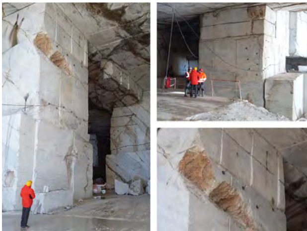
Fig. 3 - Underground areas with installed reinforcement bolts
