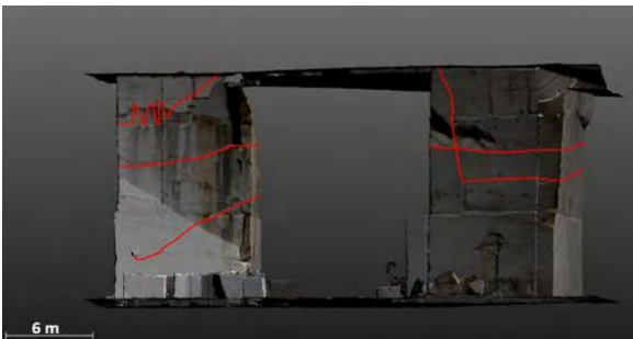
Fig. 8 - Perspective view of the texturized 3D model (mesh type) of the pillars; the red polyline represents the DOFS installed on the column sides
