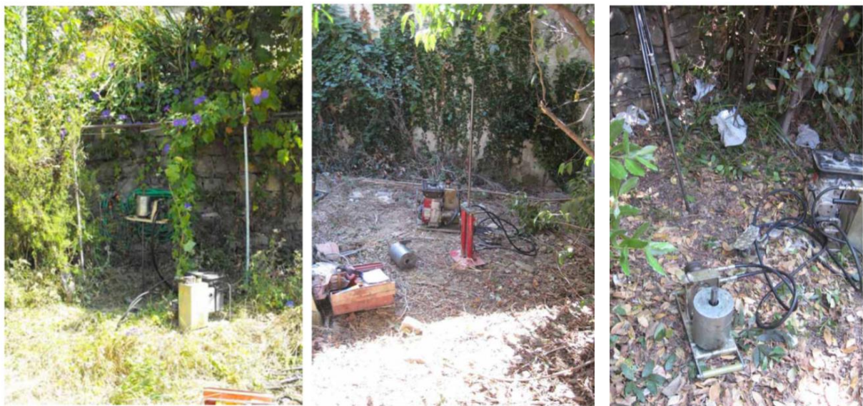
Figure 5.6 Photo of three dynamic penetration test, respectively DP3, DP8 and DP9
