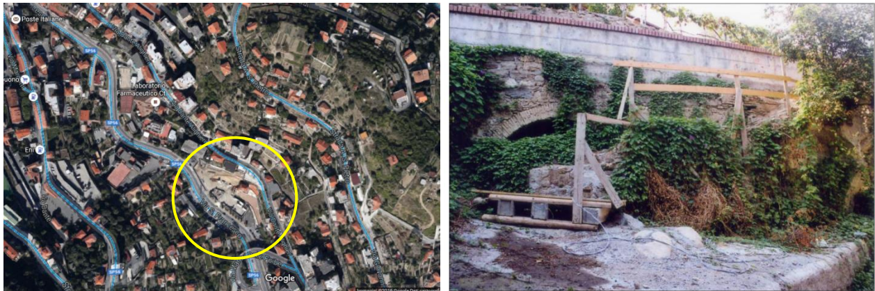
Figure 5.4 Google map view (left), photo of rock outcropping along the San Francesco torrent (right)
